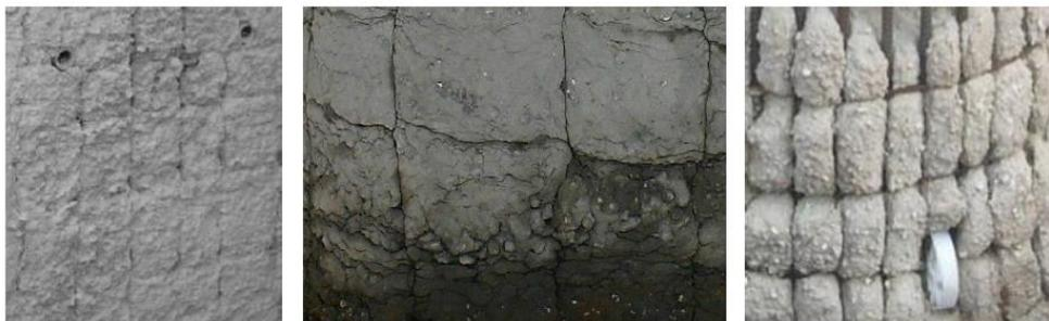
Figure. 1.5. Matting defect examples (EFFC/DFI, 2018; Bowen, 2013; Mullins et al, 2005)
