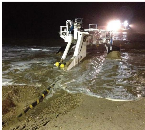
*Figure 6: Cable plough beginning operation at the shore [4]*
