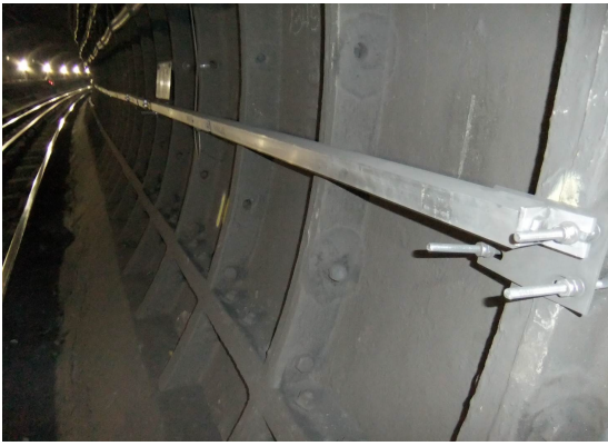
Fig. 4.1 (a) Bakerloo NB Electro-level Beams (EL Beams 14-9) [59]
