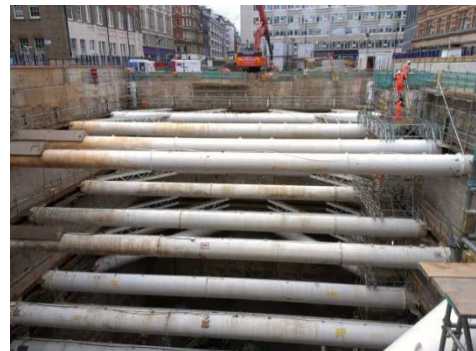
Figure 1.3.1 Dean Street Excavation (September 2012)
