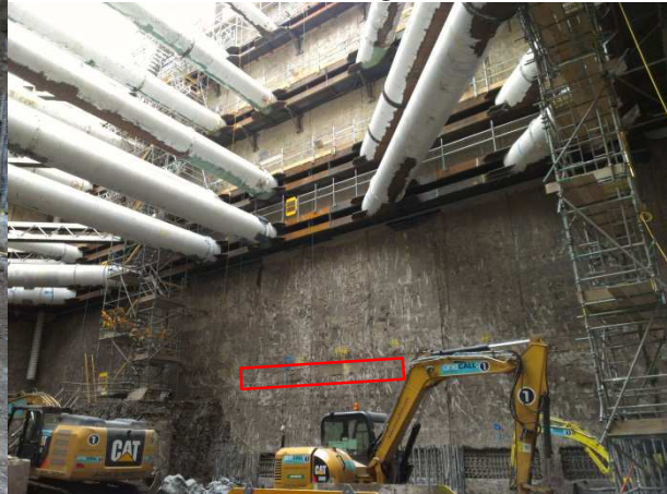
Figure 1.3.4 Fifth Prop Location (September 2012)
