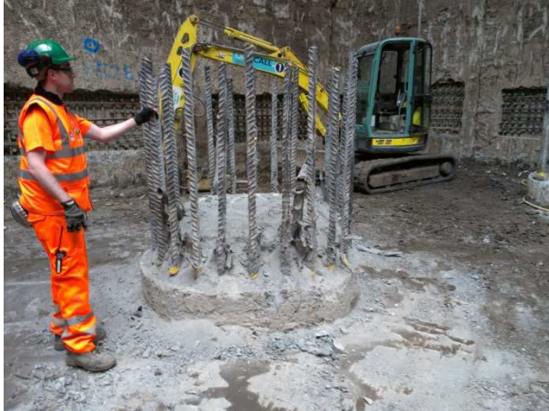
Figure 1.3.4 Cut Piles (September 2012)
