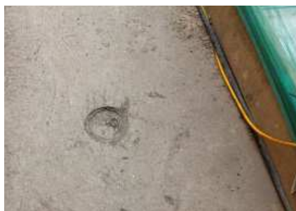
Figure 1.3.2 Primary Circuit Pipe on the top of Dean Street
