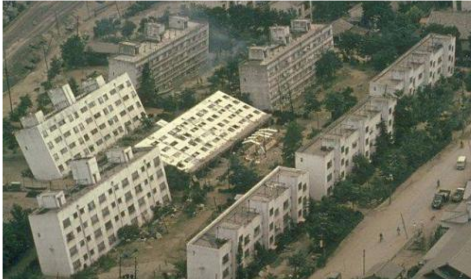
Figure 1 - Effects of Liquefaction Following 1964 Niigata Earthquake
