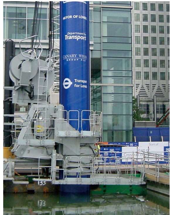
Figure 2: Suitable for use on marginal sites: a pile-jacking machine sitting atop previously installed piles in the docks in Canary Wharf
