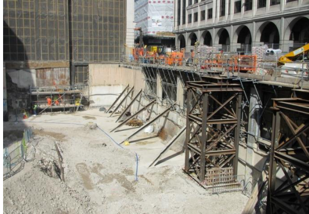
Fig 1.2 Current Bevis Marks site (March 2012)
