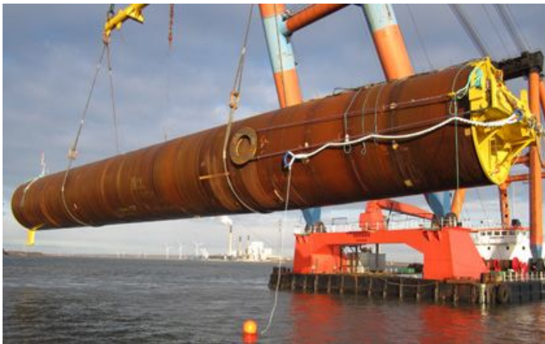
Figure 1.4: A 5m diameter, 45m long monopile ready for installation at the Anholt wind farm (Photo: DONG Energy, 2012).
