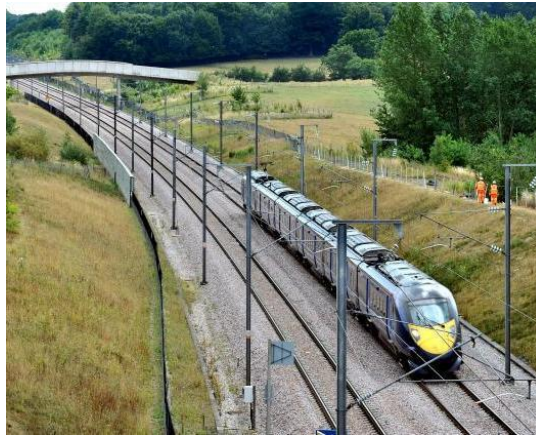
Figure 1.2 High Speed 1 Rail
