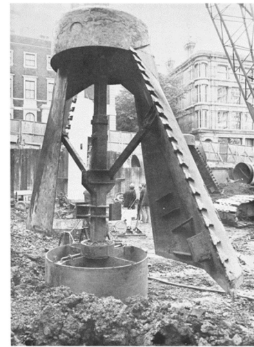
Figure 3: Top-hinged under-reaming bucket (Tomlinson, 2001)
