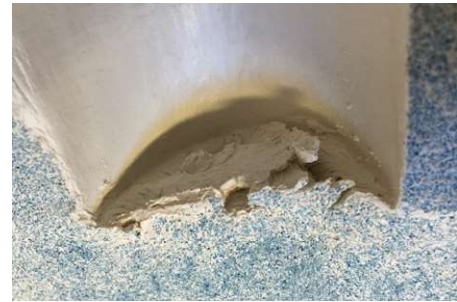
Figure 28: Evidence of base suction
