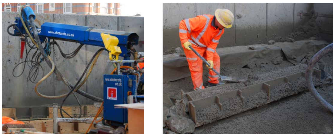
Figure 4.5 Spraying and finishing
