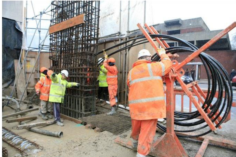
Fig. 4 - Geothermal loop at Bulgari Hotel(T. Amis, 2010, Bibliography [6])
