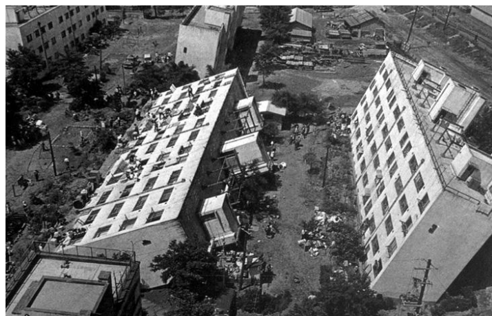
Figure 1 - Sinking of 'heavy' structure - Niigata, Japan 1964
