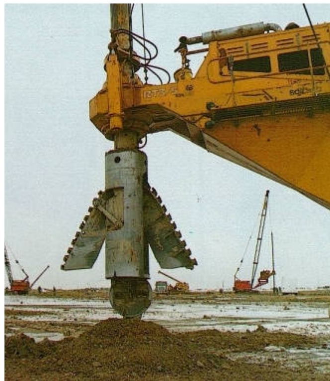
Figure 2 Under-ream excavator being emptied, geoforum.com (2009)
