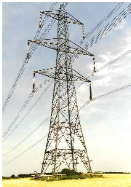
Figure 1 A transmission tower that could experience wind loading leading to uplift forces on the foundation, Savory (2009)
