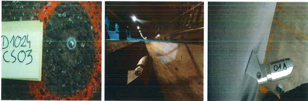
Figure 3-5 - Ground Pin and Mini Prism Installation Photographs
