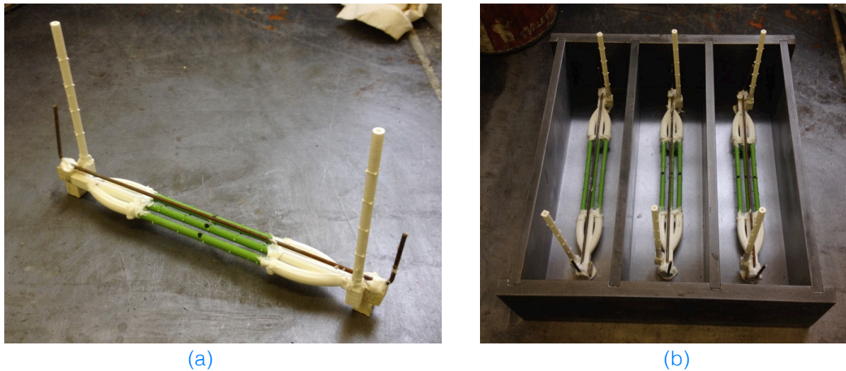
Figure 12: (a) The full assembly of network, reinforcement and ceramic spacers ready to be embedded. (b) Moulds ready for casting.
