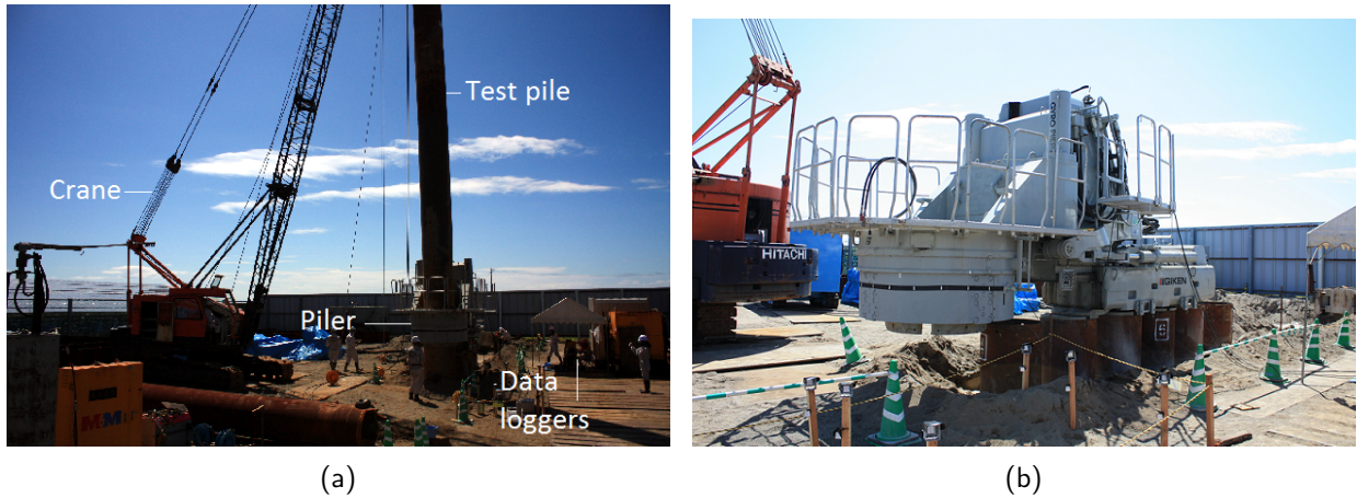
Fig. 2-3: The piler and indicative distances between the test piles.
