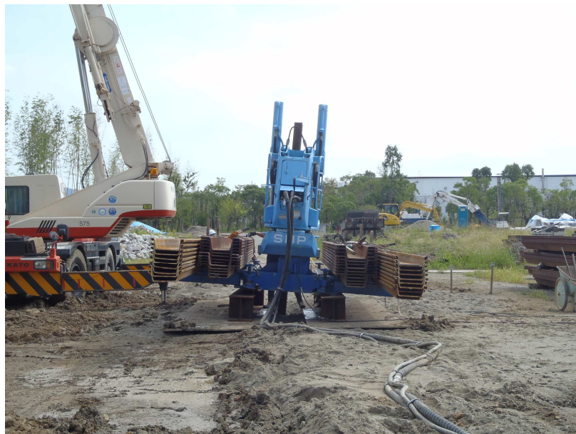
Fig.6 Installation of Slanting Wall
