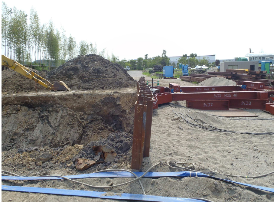
Fig.7 Preload of IP wall
