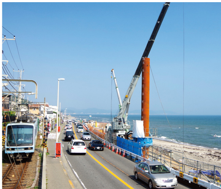
Figure 3: Steel pile walls. Elevation view (left) and Installation procedure(right)
