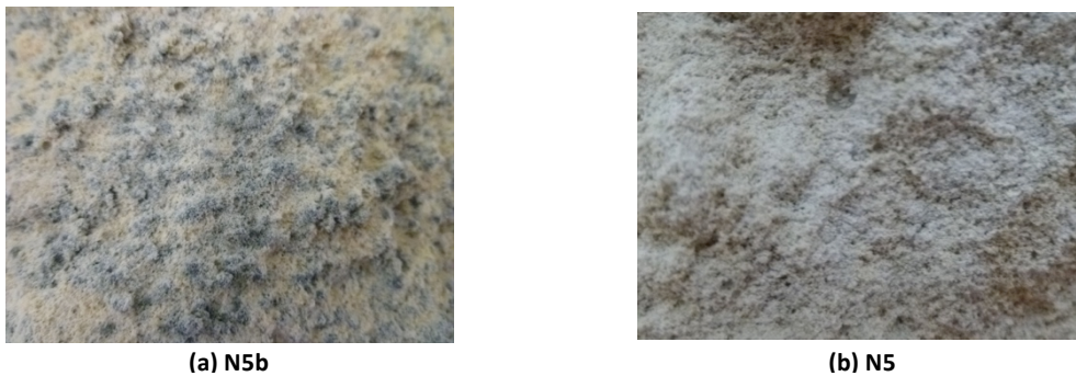
Figure 35: Close up of internal structure
