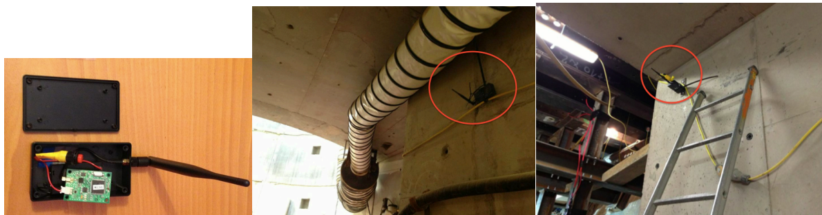
Figure 9.14: a) Left: Relay node, b) Middle: Installation of Relay node in Pal 16, c) Right: Installation of Relay node in Pal 16
