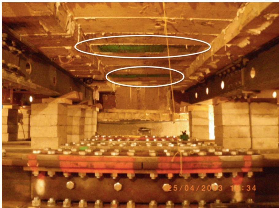
Figure 6.8: Completed temporary work (Pal 16/18 – Victoria Station); Instrumented planks circled
