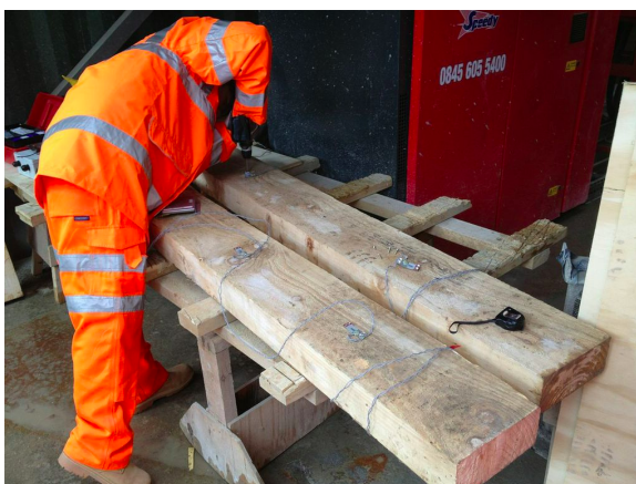
Figure 9.9: Instrumentation of plank on site
