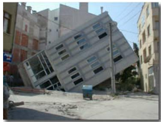
Fig. 1.1 - Foundation failure following liquefaction
