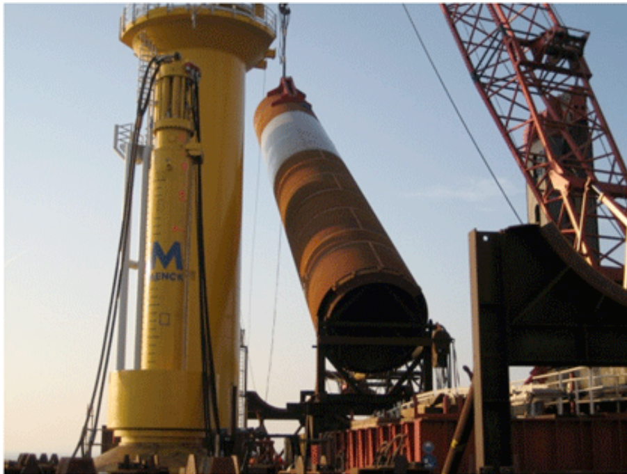
Figure 1.3. Monopile foundation pre-installation (Dong Energy)
