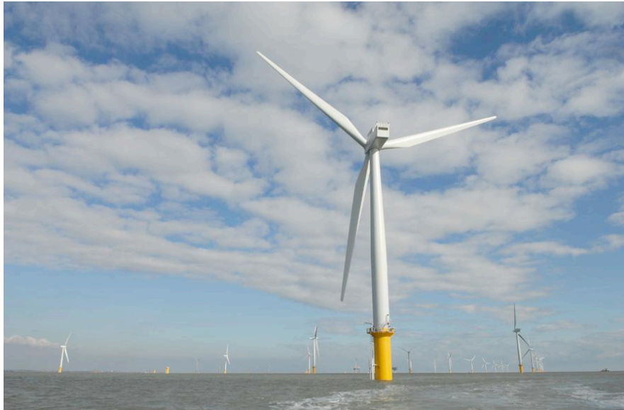
Figure 1.1. Gunfleet Sands Wind Farm (Dong Energy)
