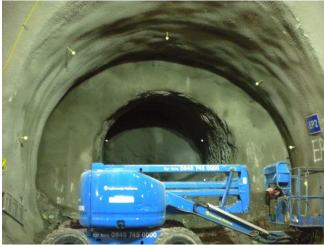
Figure 6.2.1: Example of Crossrail pilot and enlargement SCL tunnelling.
