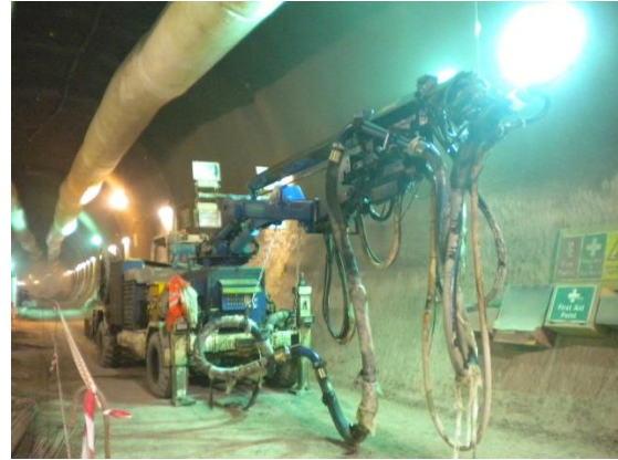
Figure 2.1.1b: Crossrail robotic SCL machine.
