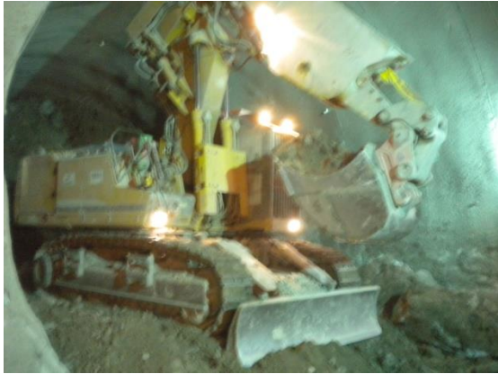
Figure 2.1.1a: Backhoe excavation of SCL tunnel on Crossrail project.
