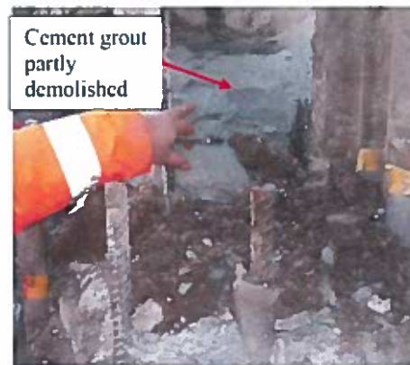
Figure 1.4: Aggregate-deficient zone [4]
