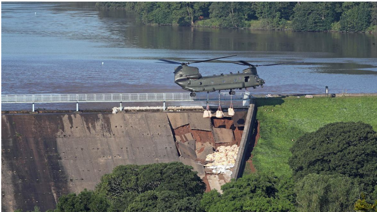
Figure 1: Chinook helicopter used to airlift aggregate on to the damaged section of the dam near Whaley Bridge
