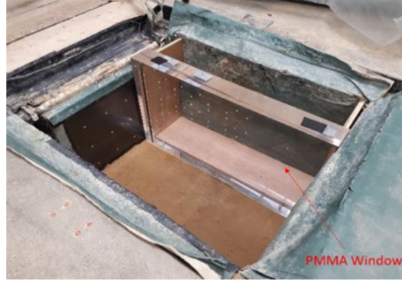
Figure 11: Installed perspex window
