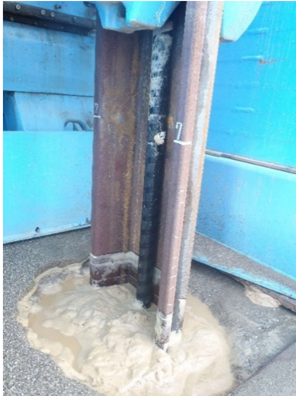
Fig. 24 Image taken during site testing showing silt particles suspended in water rising from the piling borehole (Giken, 2017)
