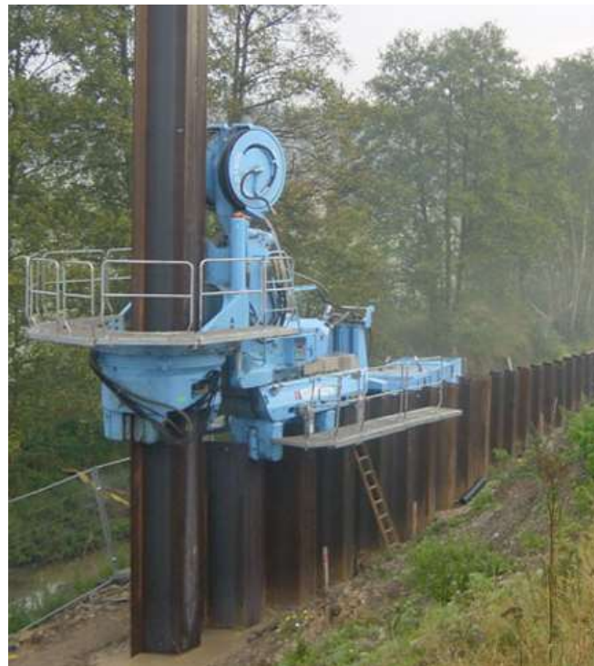
Fig. 1 Photograph of Giken’s Silent Piler installing sheet piles (Giken Europe, 2013)
