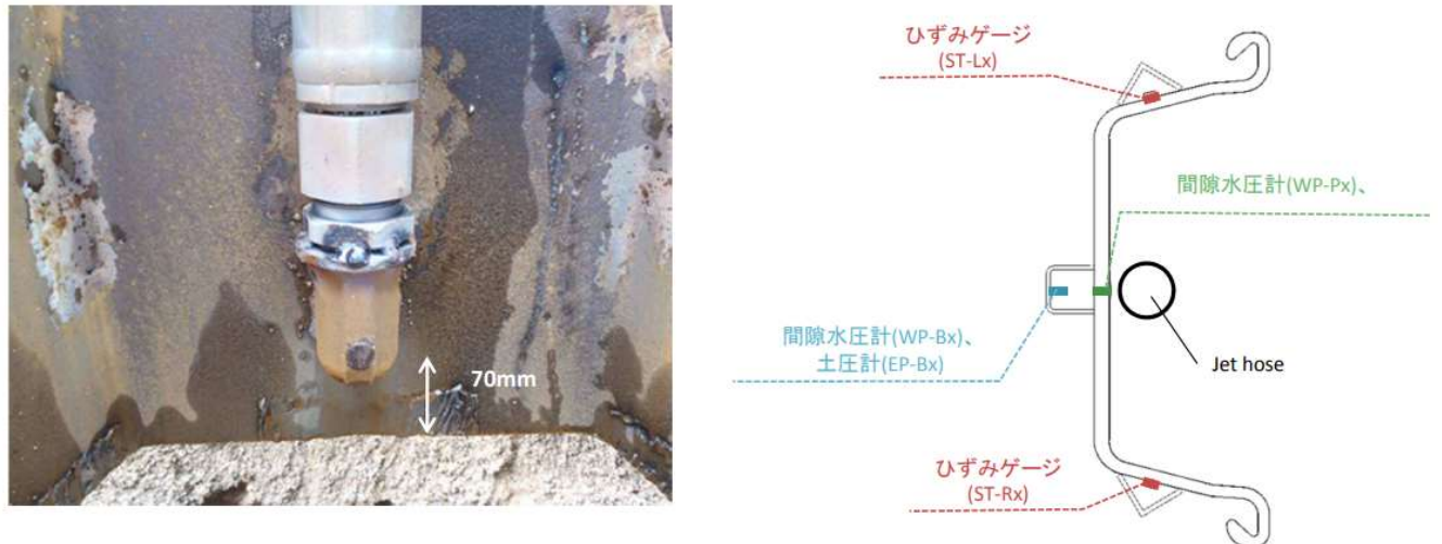
Fig. 7 Photograph and schematic showing the location of the hose at the pile base relative to the sensors (Giken, 2017)
