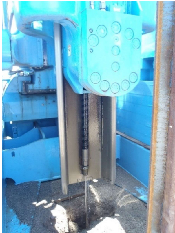
Fig. 23 Image taken during site testing showing a clean and polished pile on extraction of test No.21 (Giken, 2017)
