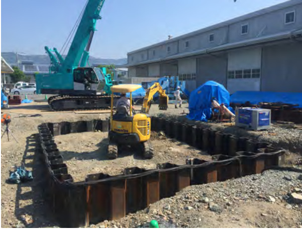
Figure 13: Sheet pile pit on site
