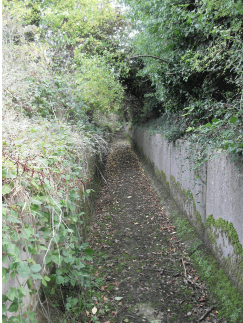
(a) Diversion channel, concrete section
