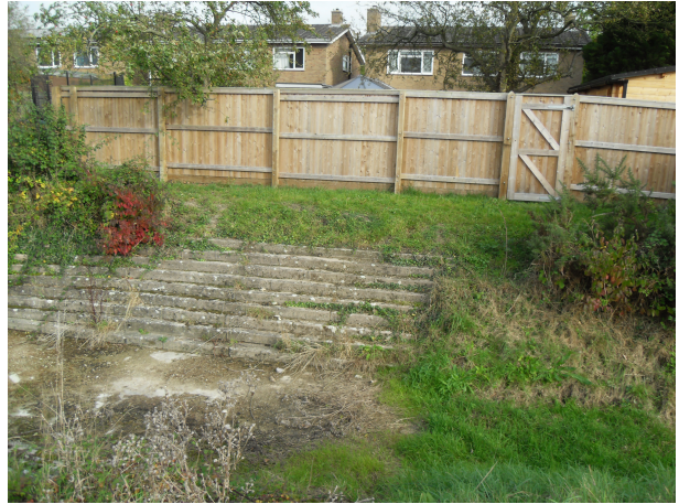
(b) Diversion channel, earth section
