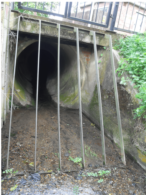
(c) Gough Way culvert inlet
