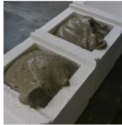
Figure 7: Foamed concrete at time of pouring, before floating.
