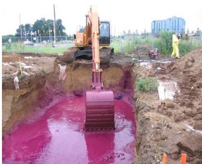
**Figure 4:** In-situ Chemical Oxidation (ISCO) Project (Reference)
